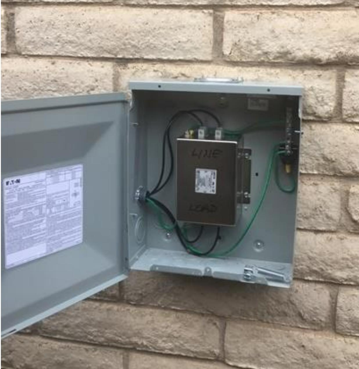
*AC unit power line filtering*
